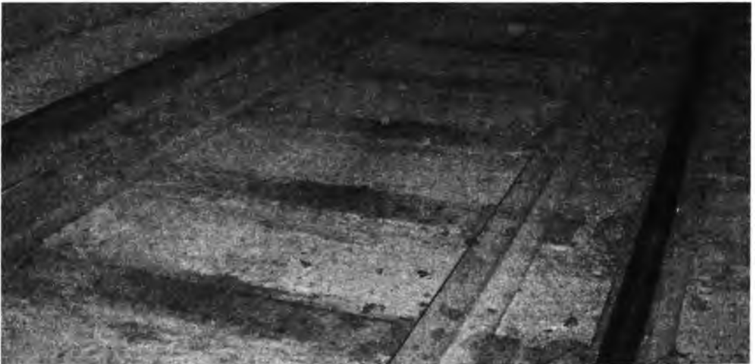
Photo 14: A view of ballast less railway track in tunnel
