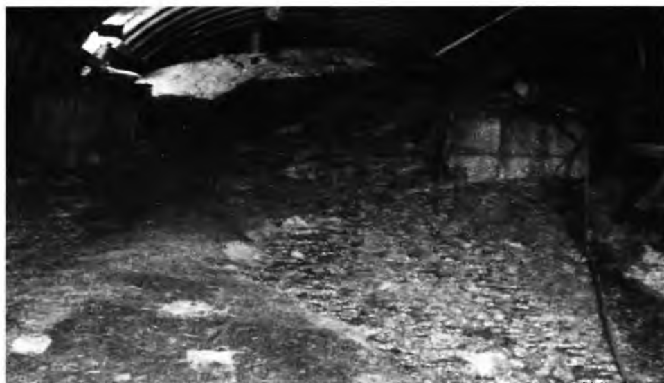
Photo 10: Crushed Dolomite with water flow in tunnel in J&K (KRCL)
