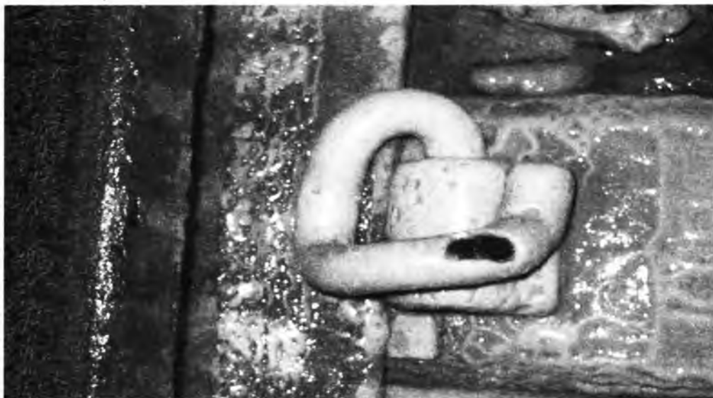
Photo 15: Damage to railway track fittings with water
