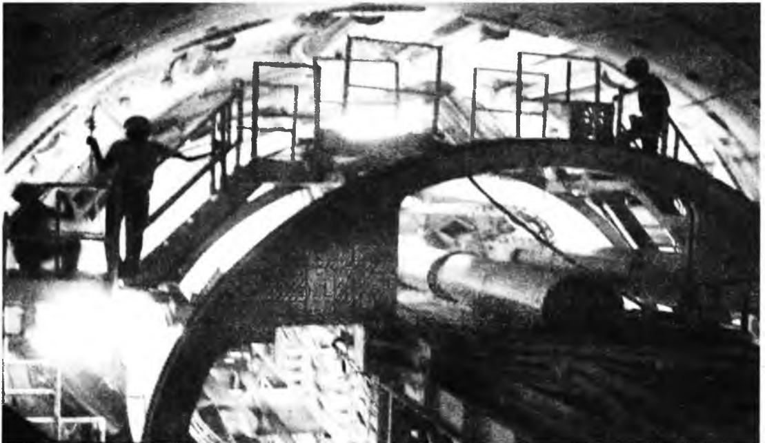
Photo 12: Tunnel Boring Machine at work in irrigation tunnel
