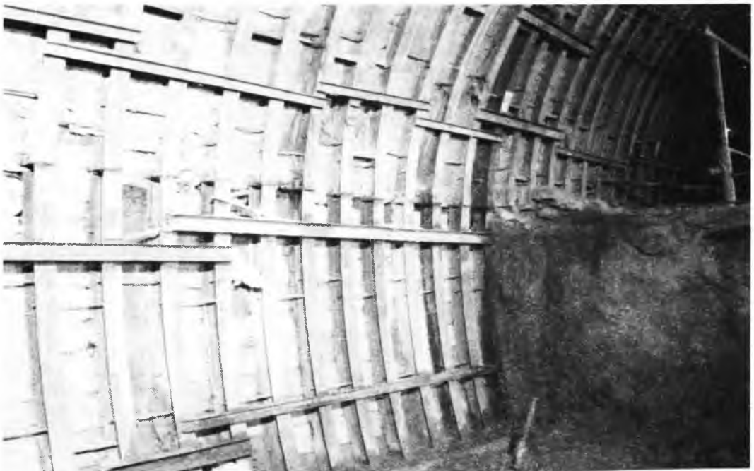
Photo 11: Drill and Blast tunnel with Heading and benching and Conventional Supports in J&K (KRCL)
